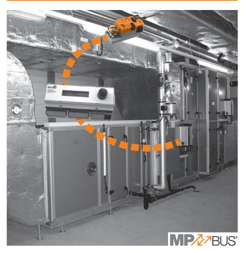
VAV/CAV system solution for energy-optimised fan regulation for room ventilation
