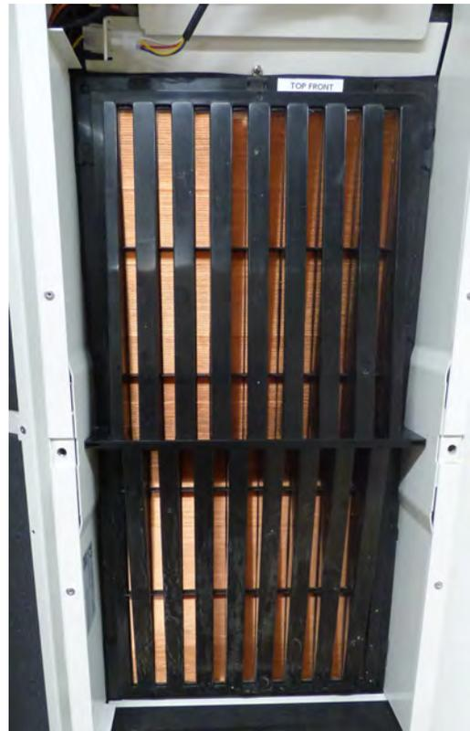
*Figure 6 – Heat exchanger ready to be removed*
