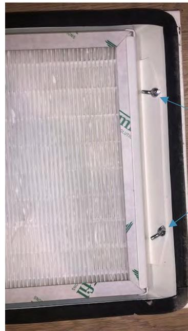
Wing nuts holding filter brace
