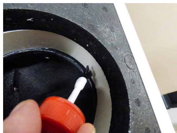
Figure 20 Use plenty – move fast as it sets quickly like contact glue
