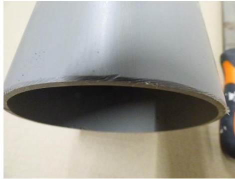
Figure 17 Deburr and chamfer the duct pipes making insertion into the white ring possible
