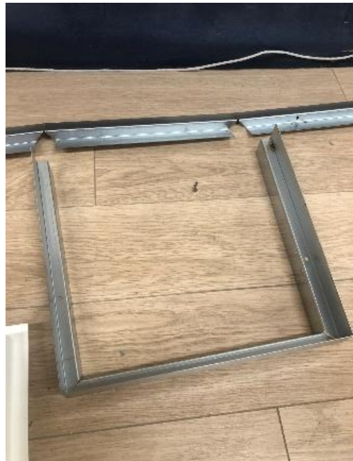
Figure 3 Bending U shape top and bottom metal edge
