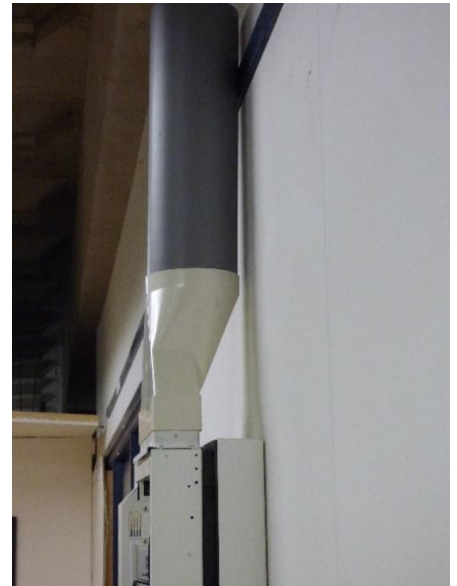
Figure 33 Square to round adapter with 125mm round connected – side view
