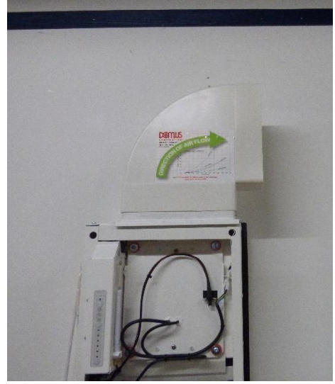
Figure 31 Low loss bend fitted directly onto adapter
