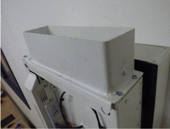
Figure 32 Fresh-r standard duct adapter 204 x 60mm
