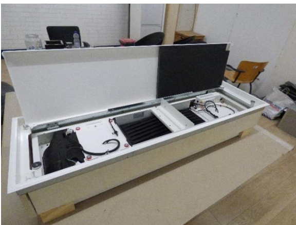
Figure 43 Fit door and frame into installation frame
