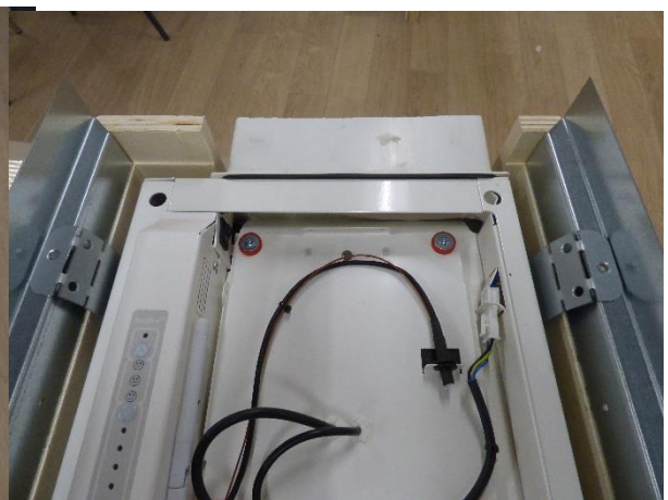
Figure 28 Fresh-r everywhere mounted inside installation frame
