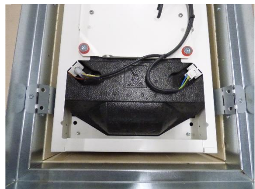
Figure 26 Lower end of fresh-r properly secured
