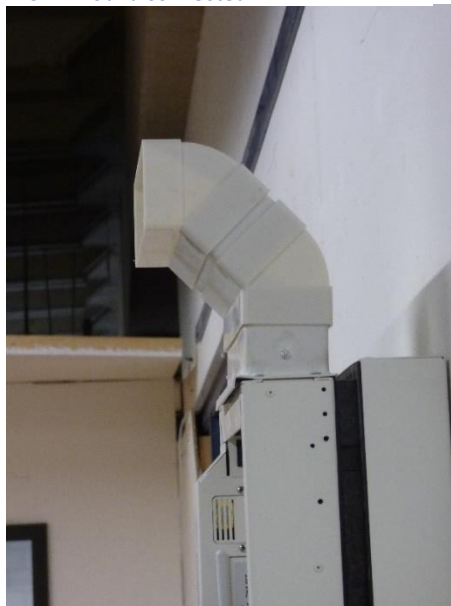
Figure 37 90 degree bend using 2 X 45
