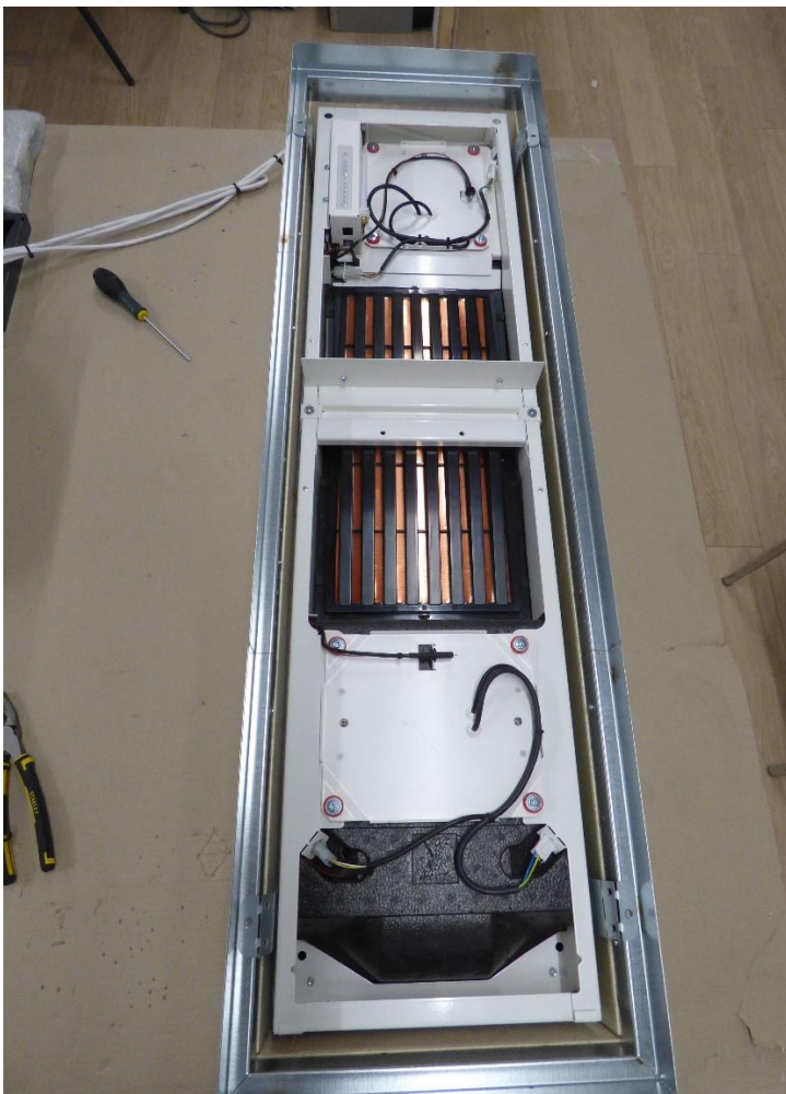
Figure 30 Fresh-r mounted inside installation frame
