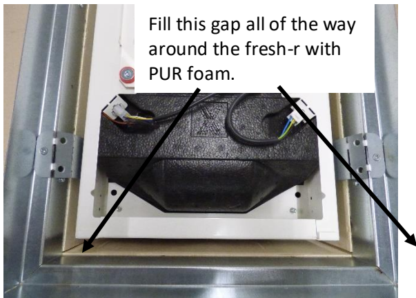
Figure 41 Insulate between fresh-r and installation frame
