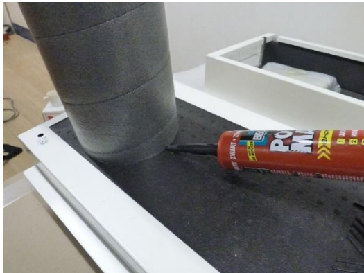
Figure 24 Internal wall sealing
