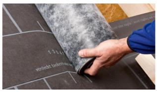
**2. Overlap the membranes** Allow for an overlap of approx. 10 cm (4") between the membranes. The marking that is printed onto the membrane will serve as a guide here.
