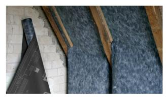
**Fastening and water flow** Affix battens at the sides. Alternative: Use DASATOP FIX. Ensure drainage through the knee wall into the eave area.
