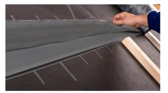
**4a. connect adhesion technology** Sticking of membrane overlaps using connect membranes with two integrated self-adhesive sections.
