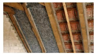
**Install the membrane** Install SOLITEX longitudinally or perpendicularly, proceeding in turn from one space between rafters to the next. Ensure that the overlaps are waterproof.
