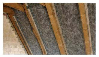
You're finished! Completed underlay retrofitted from the inside.
