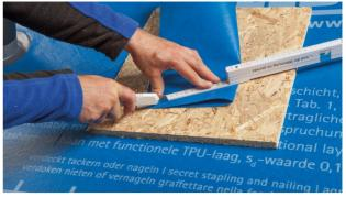
**11b. On steep roofs: Joint at pipe feed-throughs** Prepare a sealing strip of SOLITEX WELDANO-S 3000 to suit the roof pitch and pipe diameter.
