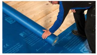
**2b. Install the membrane and overlap** Overlap the membranes at least 10 cm (4"). The printed markings are an aid to orientation.
