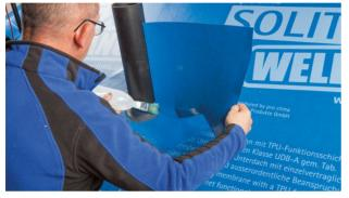
**11c. On steep roofs: Joint at pipe feed-throughs** Guide the sealing strip around the pipe and heat-weld to one another and
