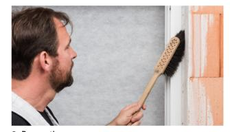
**2. Preparation** Brush off subsurfaces; if necessary, clean with a vacuum cleaner and wipe down.
