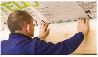
11b. Sealing to roughly sawn timber
