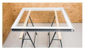
1. CONTEGA SOLIDO IQ is fitted before the window is installed
