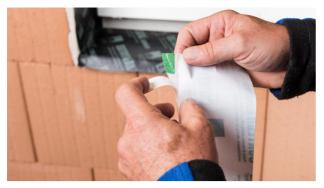
3. Removing the first release film strip
