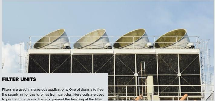
to pre heat the air and therefor prevent the freezing of the filter.
